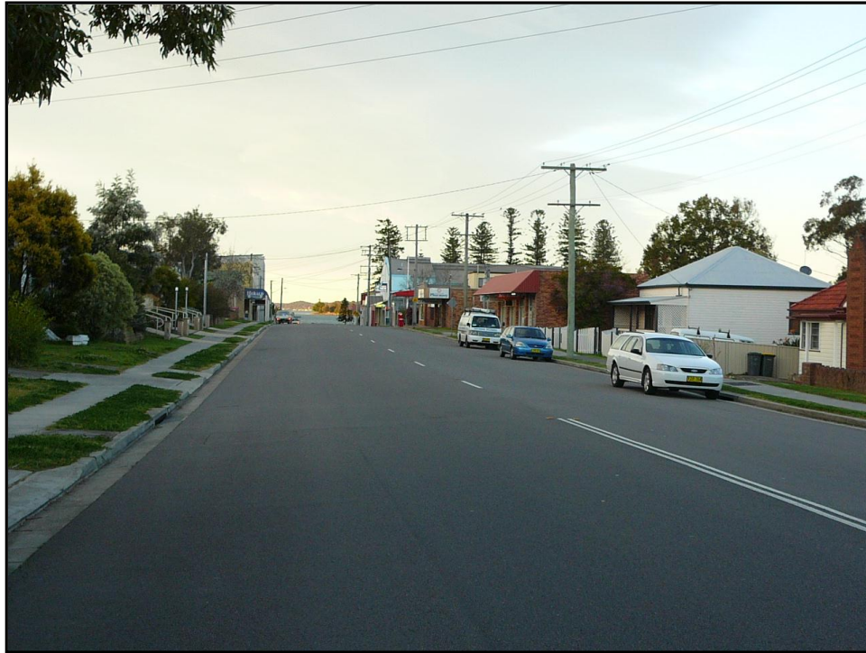
Photo 3: View south showing typical cross section on Main Road.
