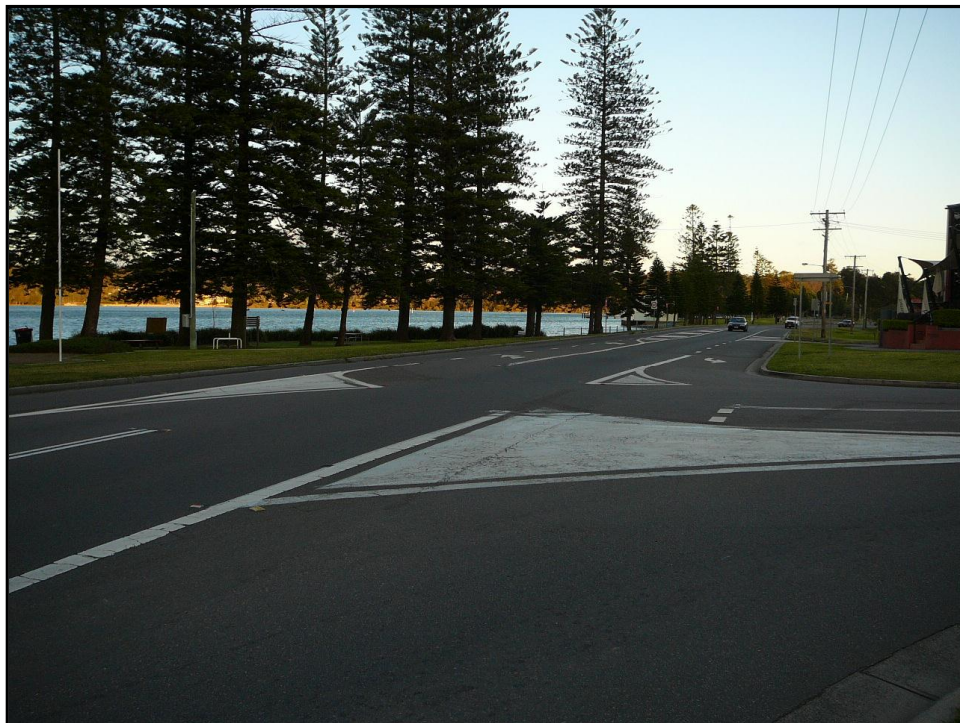
Photo 4: Layout of intersection of The Esplanade and Main Road. Note turn lanes and good visibility for drivers exiting the side road.
