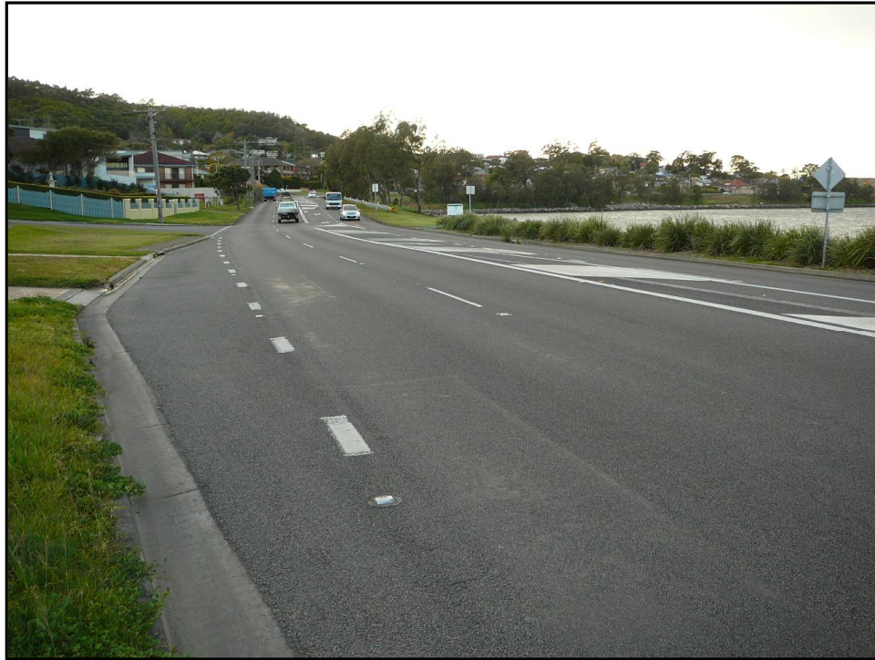
Photo 5: View east along The Esplanade showing typical cross section and layout of intersection with Albert Street.
